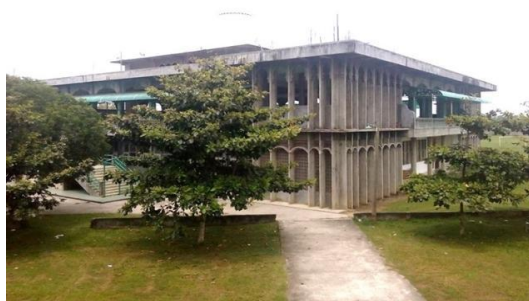
Figure 3. The building in the back yard
